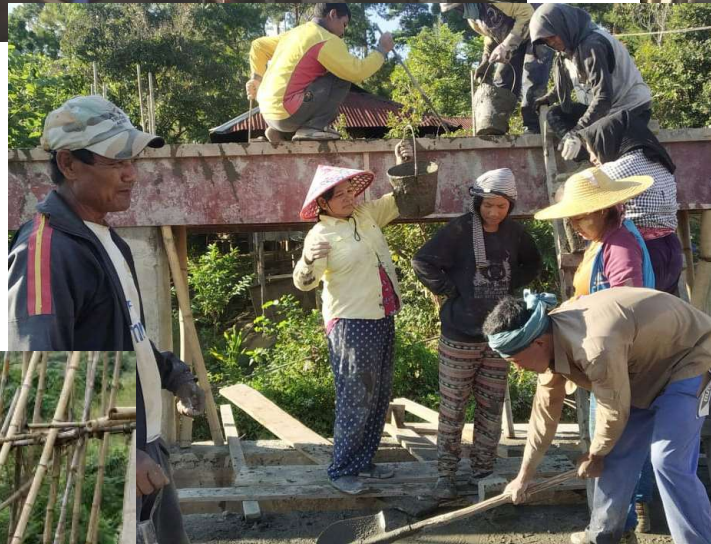
Working on the new Building in Ngoiphai.
